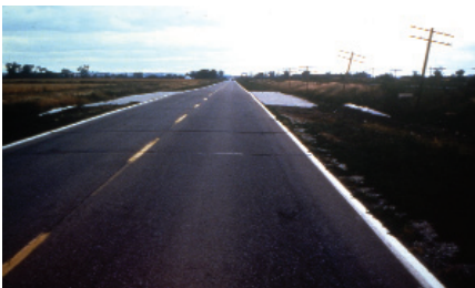
Figure 5-5. Bridge replaced by culverts and flowable fill.
