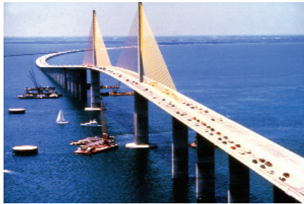
Figure 3-4. Fly ash concrete is used in severe exposure applications such as the decks and piers of Tampa Bay's Sunshine Skyway Bridge.
