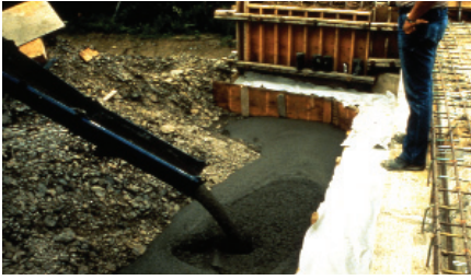
Figure 5-4. Bridge abutment backfill with flowable fill.
